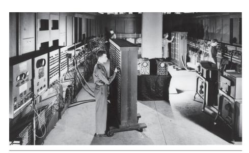
FIGURE 1.10.1 ENIAC, the world's first general-purpose electronic computer.
